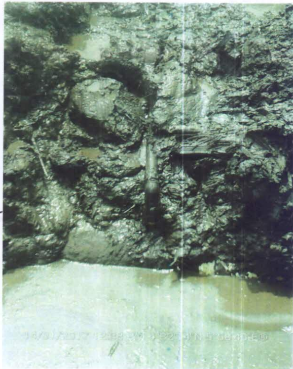
3" VALVE WITH 2" PIPE CONNECTION ATTACHED TO THE FACILITY
